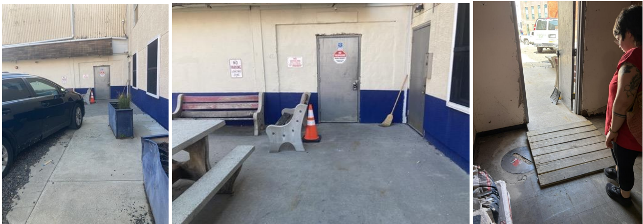
Left and center images show the accessible doorway. Right image shows inside view of accessible doorway.
